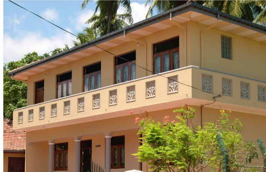
The New Building Outside
